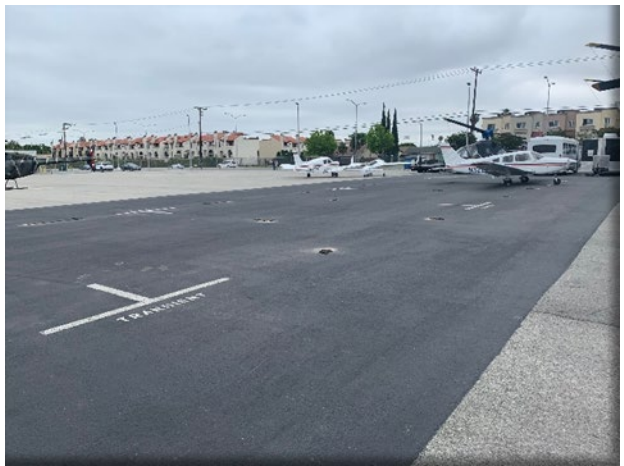
South Tiedown Area
