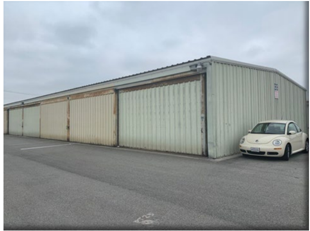
Permanent T-Hangar (Large) Row BB
